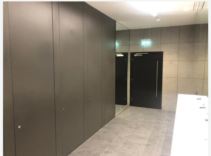
Our metal framed non-plumbed washroom panelling system, Frameduct, was specified for the WCs and urinals. The sturdy metal-framed panelling system makes for quick installation while the 90° linear bearing hinged panels offer easy ongoing maintenance. Further elevating the look of the washrooms, a bespoke herringbone design was routed into the panels.
